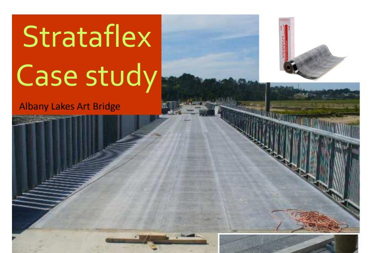
In 2008, 300 m2 of Stratflex was used to ensure a fracture free installation of the Albany Lakes Arts Bridge. Since then , no cracks have appeared in the stone or grout joints.
